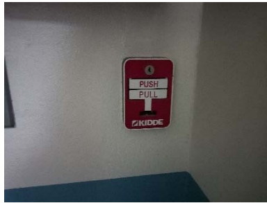
Fire Alarm Manual Station
