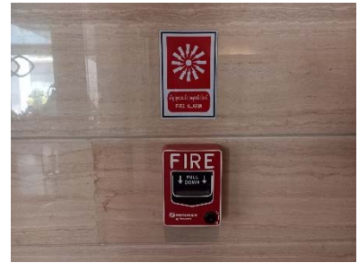
Fire Alarm Manual Station
