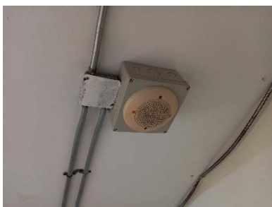
Indoor Selectable Output Speaker
